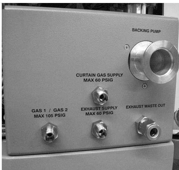
Gas and vacuum panel
